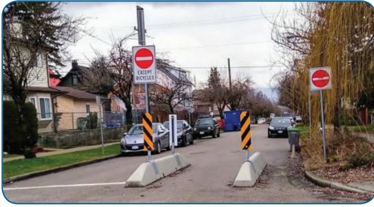
Typical slow street barrier - a temporary installation
